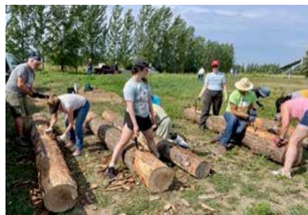
Bark stripping of building logs.
