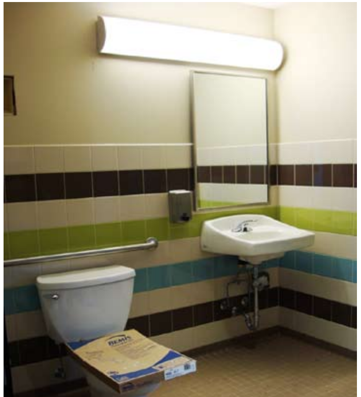
The beautifully renovated Spirit Play restroom.
