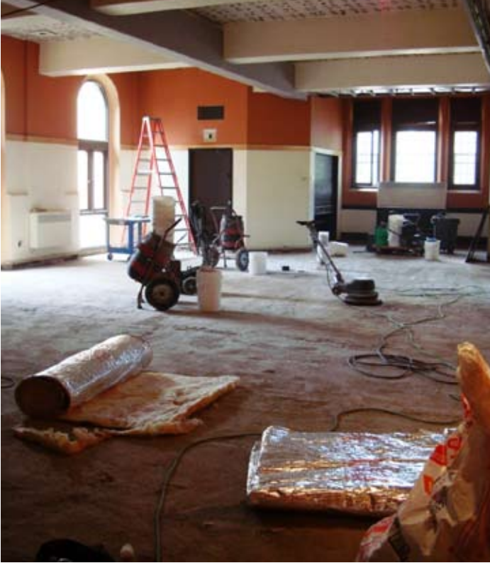
The Parish Hall floor is prepped for new hardwood.
