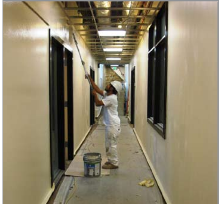
Painting at the upper level Eliot Wing.
