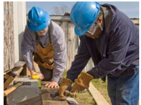
Ted Lentz and Rev. Carl Walker saw wood to begin framing.
